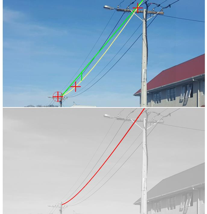
Fig. 1. Power line fitting using 3 manually selected points on the curve (top) versus our automatic power line detection method.
